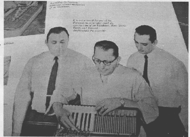
Mario, Egisto and Edward Pancotti inspect the construction of an Excelsior
